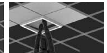
Place 2x2 ceiling tile on the luminaire
